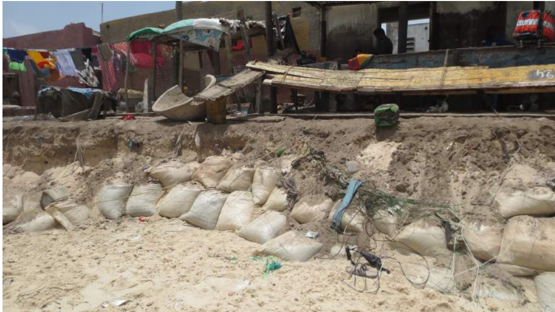
Figure 2: Sand bag barriers stabilized with old fish netting. Goxum Bacc, Saint-Louis, Senegal.
